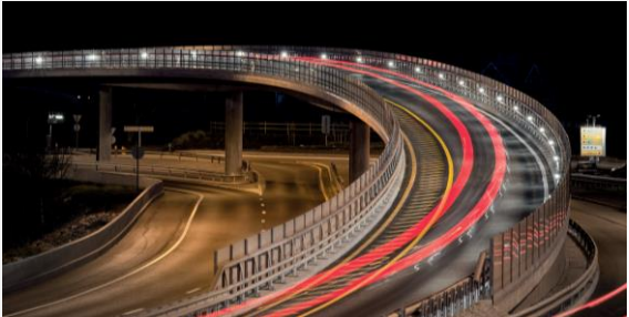
Roads, Transportation & Tunnel
